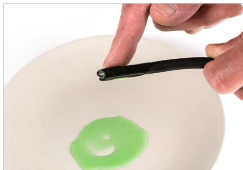
**2.2** Lubricate the cable cover with soft soap or similar product. This will ease up the process of getting the cable through the cable entry components. **Ensure that the cable is disconnected from eventual power sources.**
